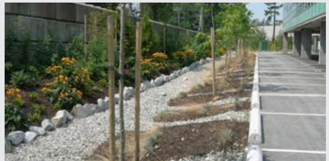
Figure 4. An Innovative parking lot in North Vancouver where runoff is infiltrated into a sand and gravel filter
