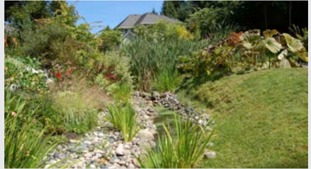
Figure 3. Rain-garden in Surrey, B.C. that allows the surface runoff to infiltrate into the soil
